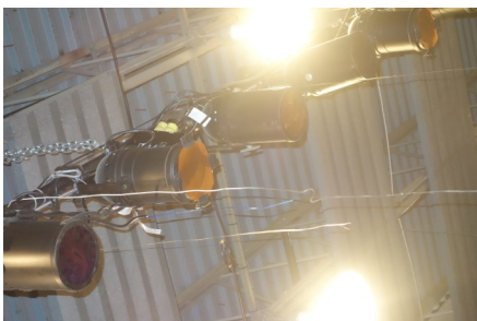
24X Par Can lighting fixtures—1000Watt 3x 24' x 1 1/2" Dead hung pipe
