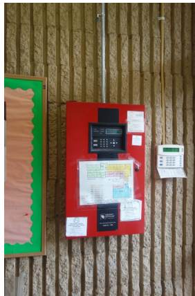
Silent Knight Alarm System Model SK-5208
