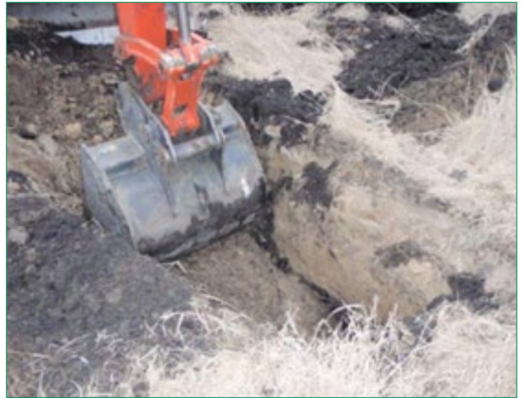
Excavation of a test trench on industrial land where soil contamination is suspected.
